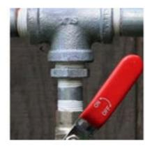
**Galvanized iron or steel.** If the pipe is silver or gray, hard to scratch with a key or coin, you may have an iron or steel pipe. If you place a magnet on the pipe and it sticks to the pipe, you may have galvanized steel pipes.
